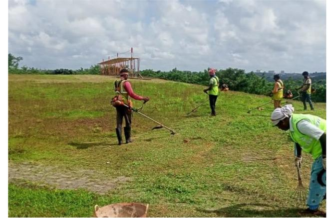
Manual hand machine deployed for vegetation control.
